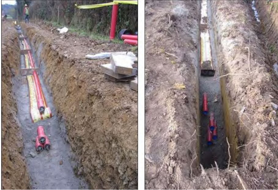
Plate 4-1 Typical Cable Trench View
