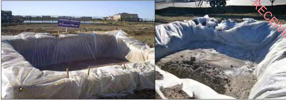
Plate 4-3 Concrete washout area
