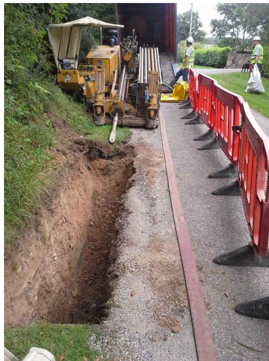
Drilling Rig & Launch Pit
