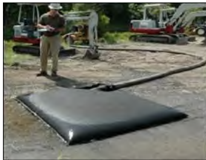
Plate 4-5 Silt Bag with water being pumped through
